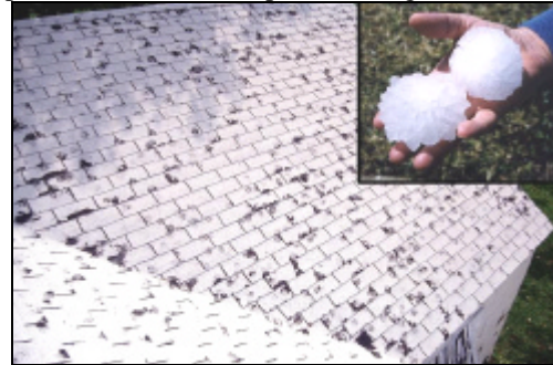
Figure 1. Hail damaged asphalt shingle roof from the Fort Worth, Texas hailstorm on May 5, 1995. Large hailstones are shown in the inset photograph.
